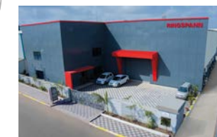
RINGSPANN Power Transmission India Pvt. Ltd., Inde
